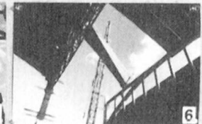
4 Lifting 40 T precast prestressed tied arch girder 30 M span. 5 Tied-arch girders erected and in position 6 6 cm thick folded plate element 12 m. 7 Folded plate elements in position
