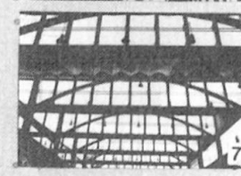
4 Lifting 40 T precast prestressed tied arch girder 30 M span. 5 Tied-arch girders erected and in position 6 6 cm thick folded plate element 12 m. 7 Folded plate elements in position
