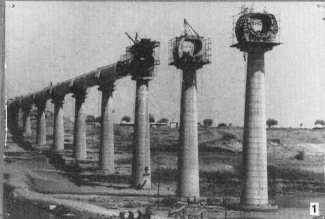
42.5 cumecs; 947 m long, 41.5 m continuous spans, 3.75 m roadway. Truncated circular cross section 4.8 m dia. Constructed by cantilever technique using epoxy glued precast matchcast voussoirs prestressed longitudinally and circumferentially.
