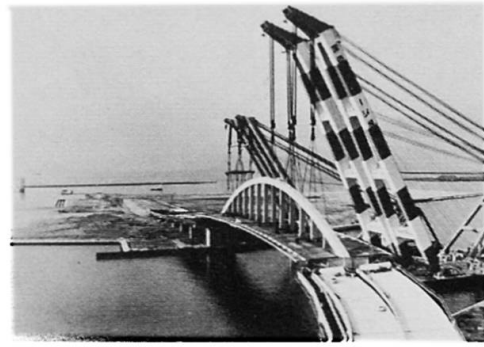
Fig.6 Izumi Otsu Bridge(1976) Span 172.572m, 3000t
