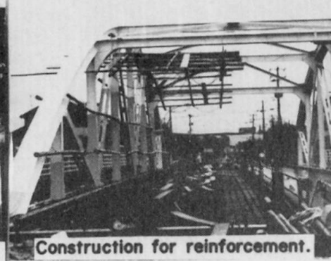
Reinforced bridge based on optimum combination of diagonal hangers.
