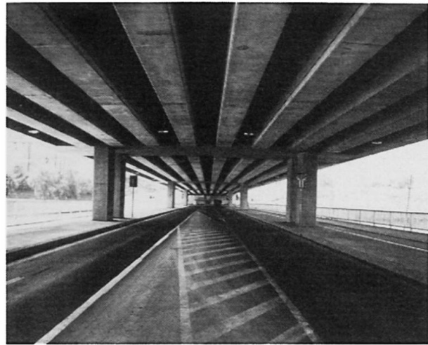
Fig. 2: The slab of the upper bridge
