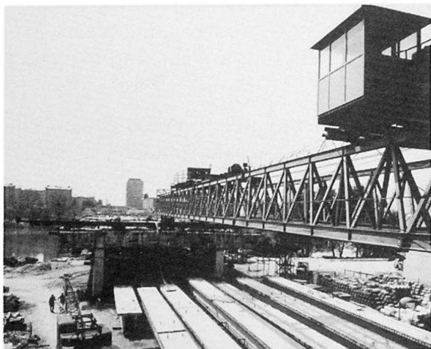
Fig. 11: Beams during grouting at the construction site.
