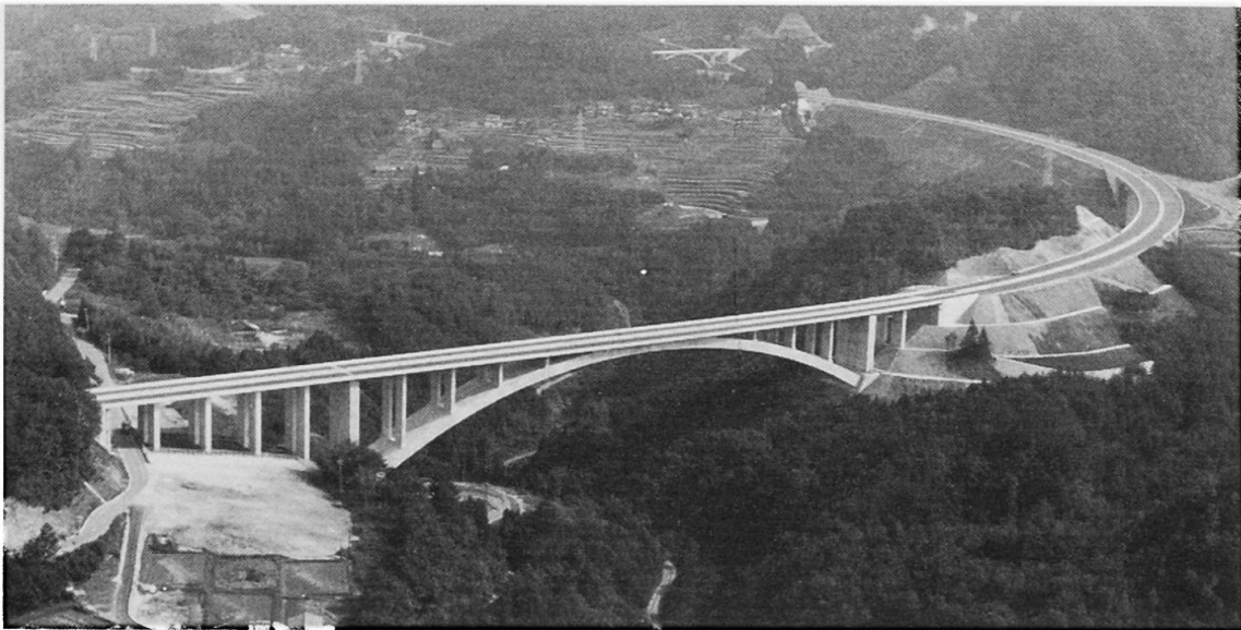
Photo 1, Appearance of Usagawa Bridge
