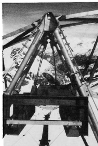
Fig. 6 Head of intermediate pylon
