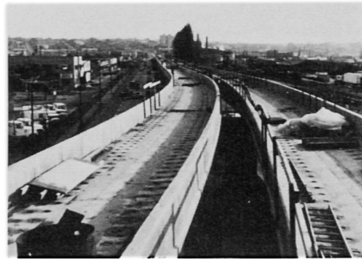
Figure 9 The Vancouver Advanced Light Rapid Transit System uses linear induction motors and continuously welded rails. Left is a photo of the completed structure from below, and right shows the beams during construction. (Photos by ABAM Engineers)
