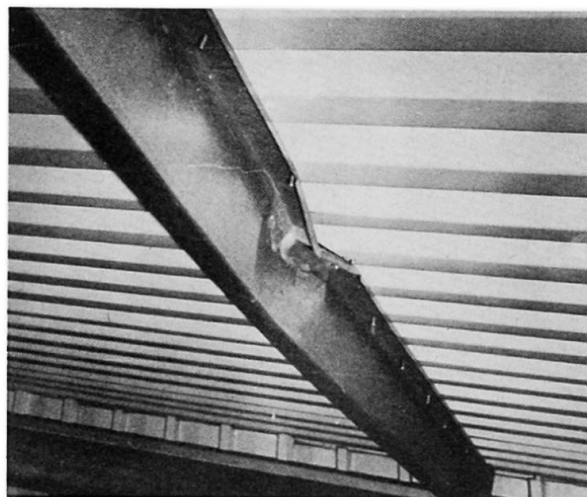
Fig.3 Buckled Z-purlin.
