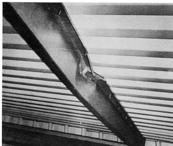
Fig.3 Buckled Z-purlin.
