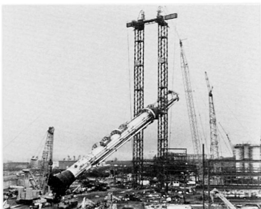
Fig. 5 Vessel Lifted 30 metres
