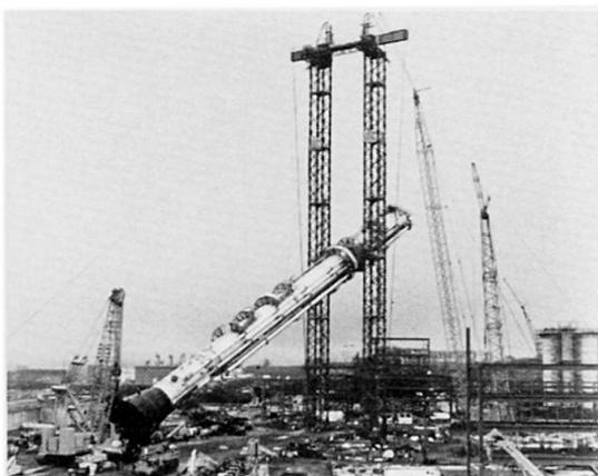
Fig. 5 Vessel Lifted 30 metres
