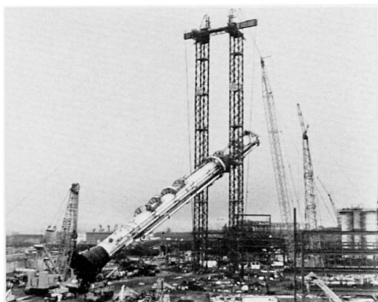
Fig. 5 Vessel Lifted 30 metres
