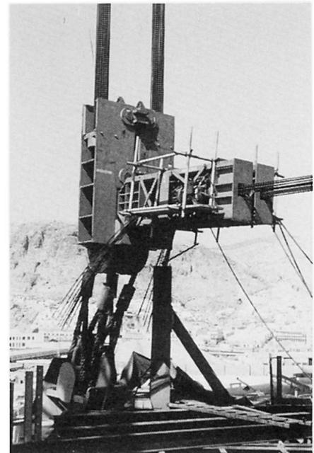
Fig. 4 Three-Way Connector.
