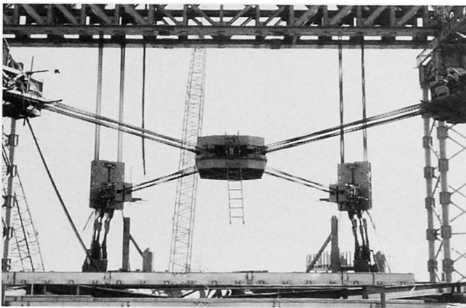
Fig. 3 Tension Frame Assembly.
