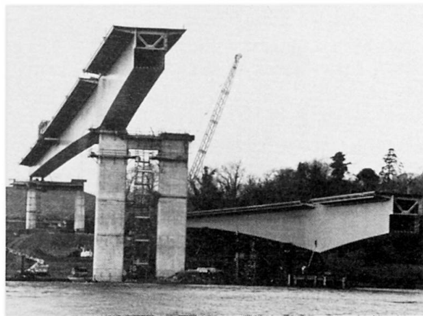
Fig. 9. Sidespan in final position
