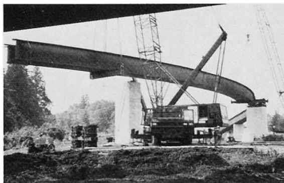
Figure 11. Girder erection.
