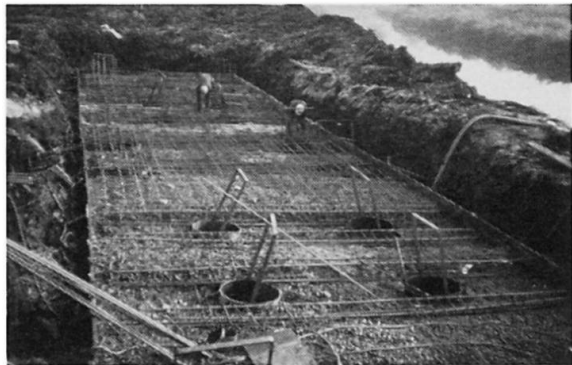
Figure 3. Pile cap working slab.
