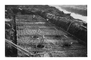
Figure 3. Pile cap working slab.
