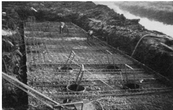
Figure 3. Pile cap working slab.
