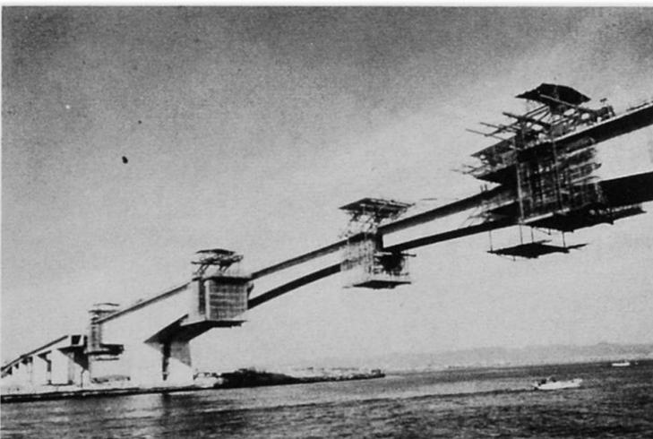
Fig. 15 Cantilevering of a prestressed concrete bridge
