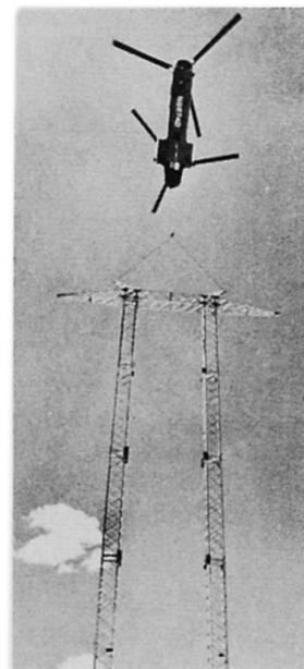
Fig. 16 Erecting a transmission tower by helicopter
