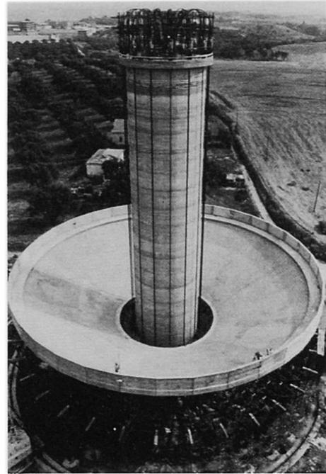
Fig. 18 Lifting an elevated reinforced concrete water tank
