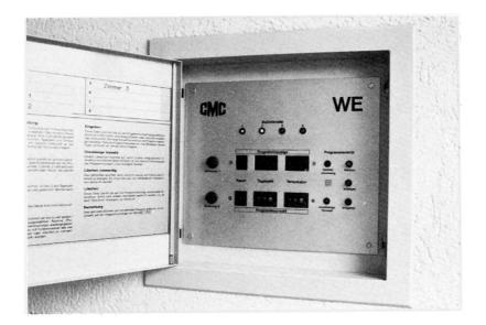
unit. It stores the information of the inhabitants programs and calculates the adjusting values for the room control valves. The supply water temperature and the deficiency heat supply (when the heat pump does not deliver enough heat) are also controlled by the central unit.
