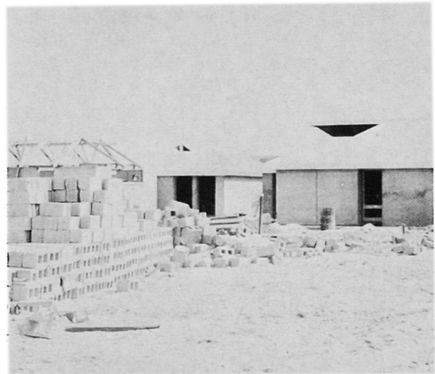
Fig.2: Photograph of typical elevation.
