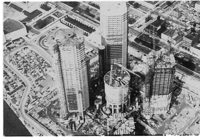
**DETROIT RENAISSANCE:** This is a very large and complex project consisting of a 70-story concrete structure hotel, four 39-story steel structure office buildings connected with a 7-story concrete podium for parking and commercial space.
