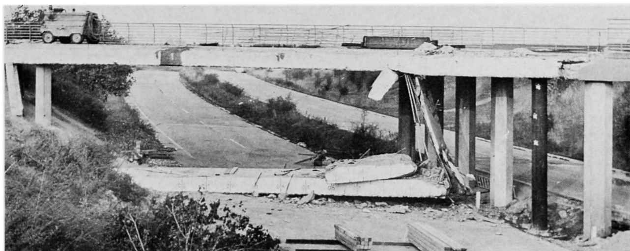
Fig. 7. The collapsed slab strip.
