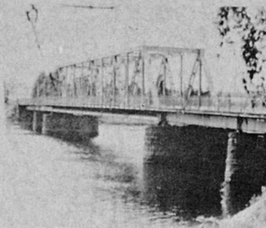
The existing steel truss bridge Spans: 70.0 + 10.4 + 10.4 + 10.4 + 10.4 m Width: 5.2 + 5.2 + 5.2 + 5.2 + 5.2 m Completed: 1925
