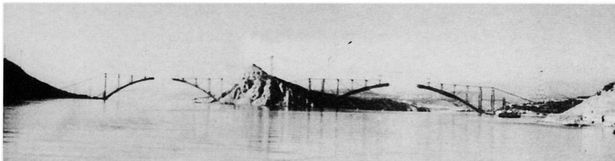
Fig. 7 - Erection of the central portion of the bridge arches
