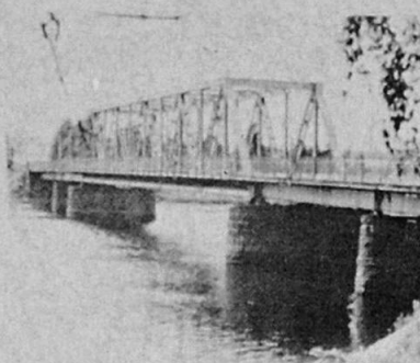
The existing steel truss bridge Spans: 70.0 + 10.4 + 10.4 + 10.4 + 10.4 m Width: 5.0 + 2.0 + 1.35 + 1.35 + 5.0 m Completed: 1925
