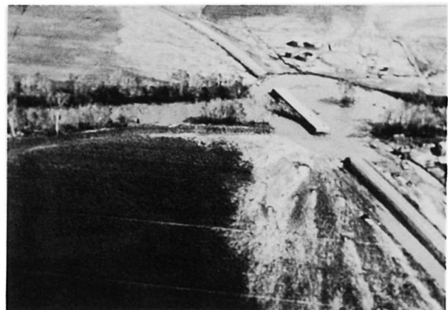
Figure 3 End scour after waterway blockage.
