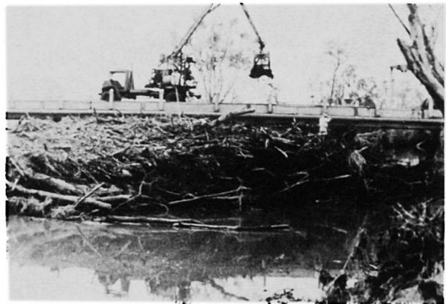
Figure 2 Spans too small Deck at flood peak
