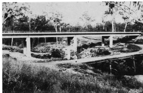
Figure 4 Submersible bridge replacing lower timber bridge
