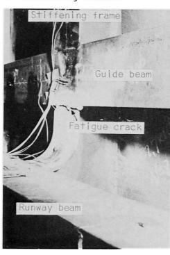
Fig. 9 Fatigue crack initiation at stiffening frame corner
