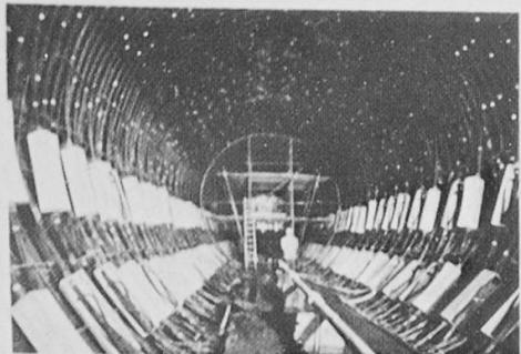
Prestressed concrete lining under construction. Pumped storage scheme, Oberaar-Grimsel, Switzerland. (Photo: Dampfwerk Unterwerke AG, Berne)
