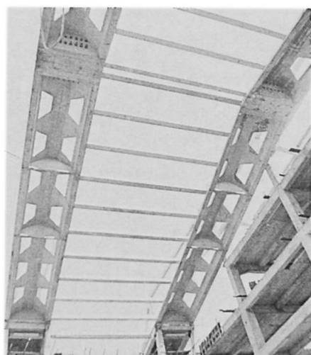
Fig.14. Inside view of the precast beam
