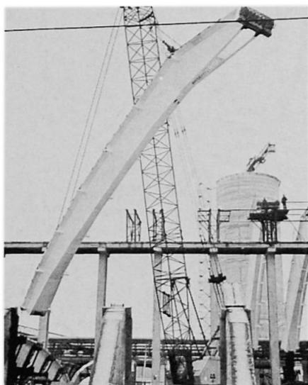
Fig.5. The handling of the precast element
