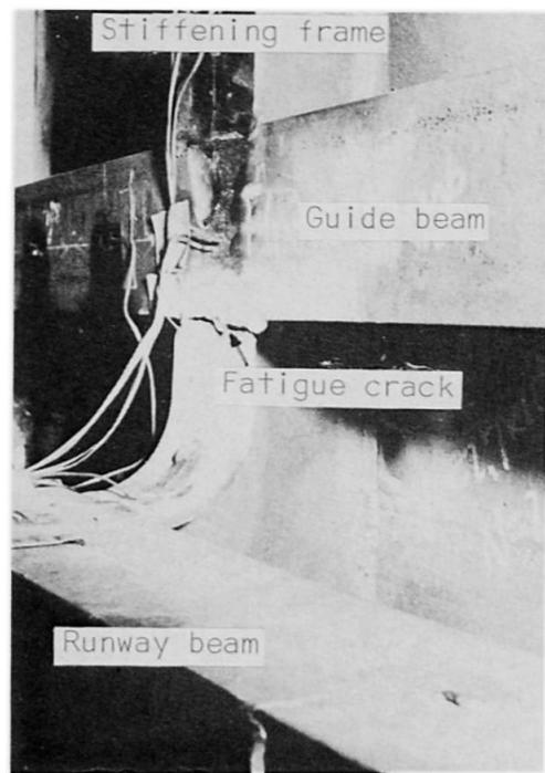
Fig. 9 Fatigue crack initiation at stiffening frame corner
