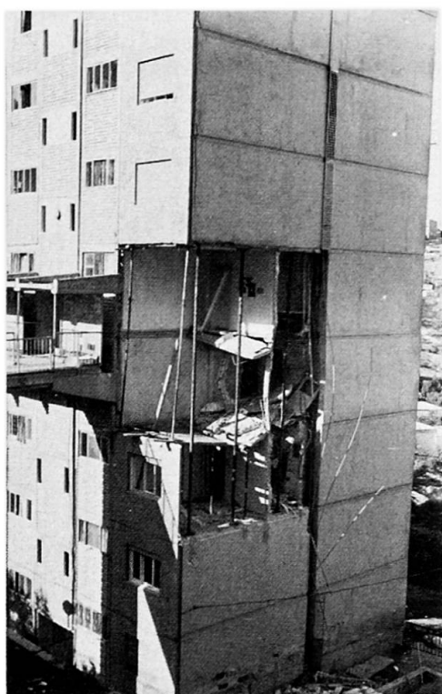
Figure (4) Results of boiler explosion in Jerusalem
