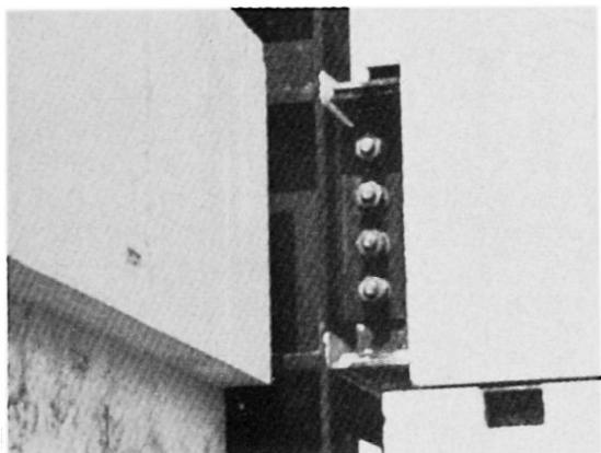
Fig. 2 Beam-column connection
