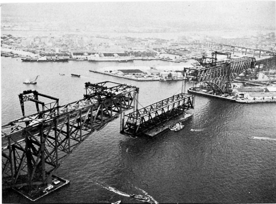
Photo 1 Lifting of Suspended Span
