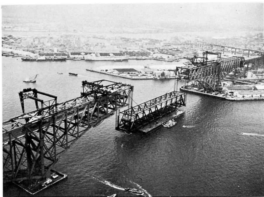
Photo 1 Lifting of Suspended Span
