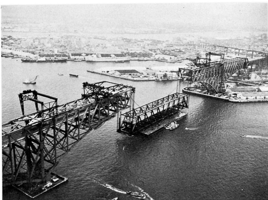
Photo 1 Lifting of Suspended Span
