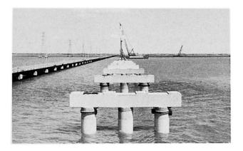
5. Newly installed piles and caps for replacement roadway
