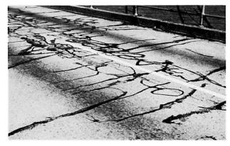
3. Deteriorated riding surface temporarily repaired with poured asphalt
