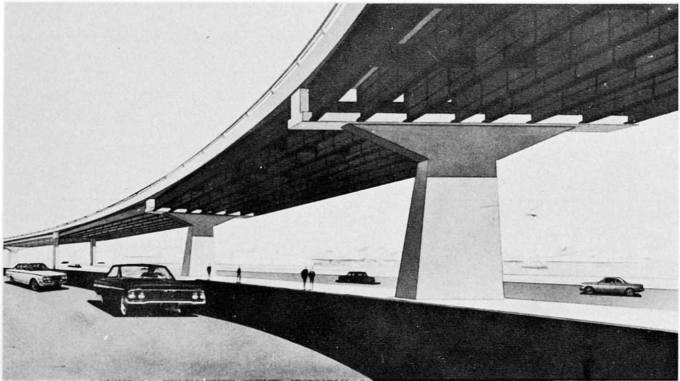
The above photographs refer to solutions with spans close to 40m and a width of the roadway of 20m.
