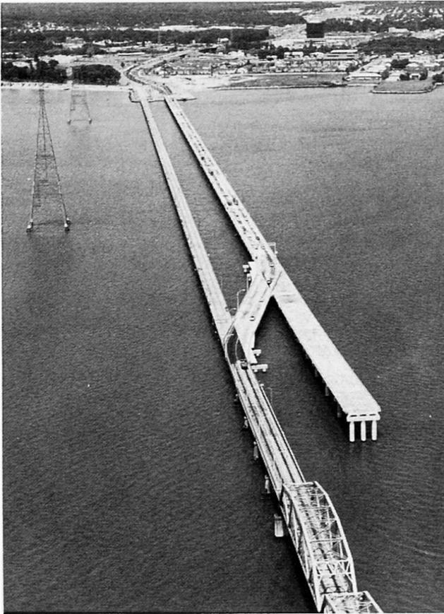
7. Old and new bridges shown during construction with crossover in operation
