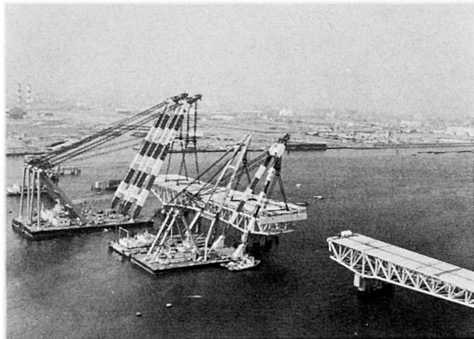
Fig. 3 Erection of the largest block (4,250 ton)
