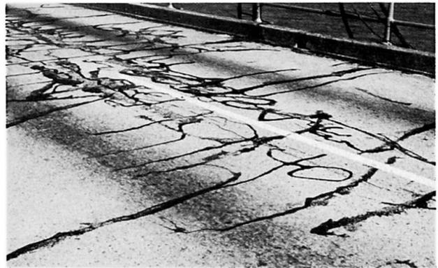
3. Deteriorated riding surface temporarily repaired with poured asphalt
