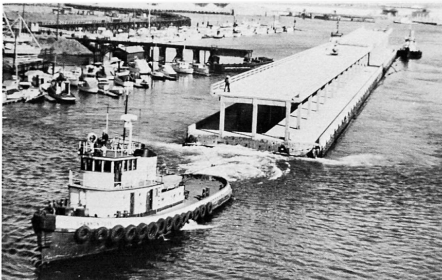
Fig. 11: Precast pontoon under tow to elevated super-structure construction site.
