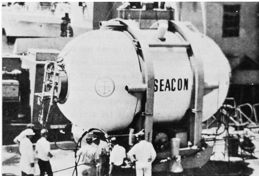
Fig. 8: SEACON, tested at 180 m below sea level by the U.S. Navy.
