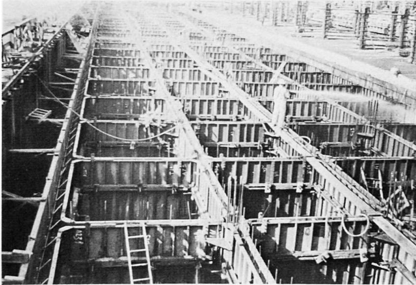
Fig. 10: Precast pontoon construction in graving dock.
