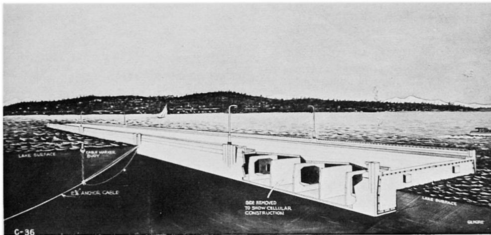
Fig. 9: Cutaway view of floating bridge pontoon.
