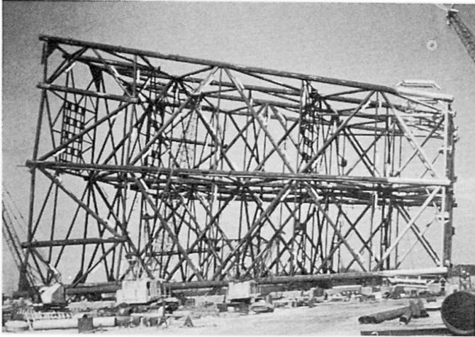
Fig. 13. Jacket at fabricating yard
