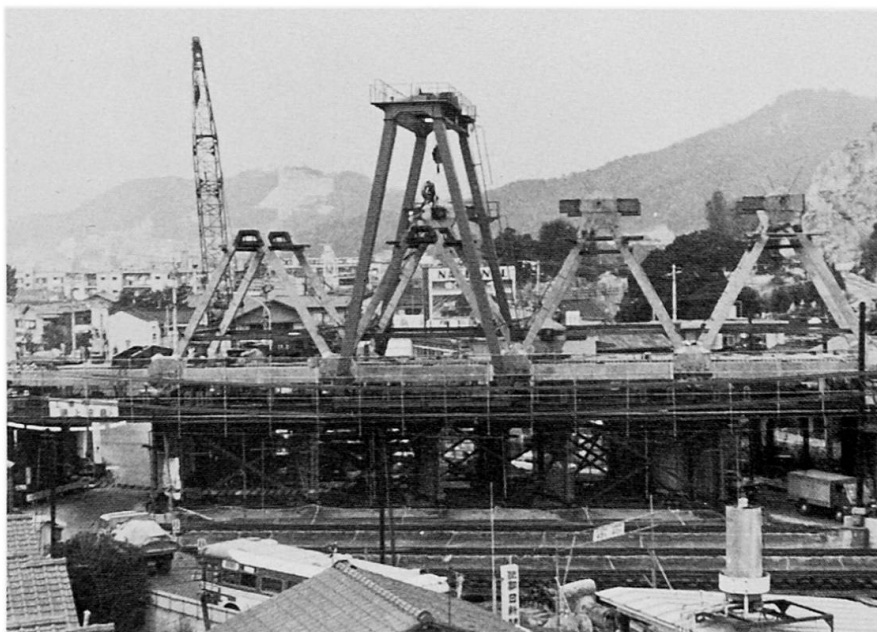
Photo 2. The Iwahana Bridge, erected on the staging
