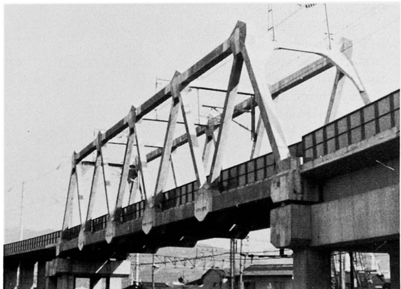
Photo 1. The Iwahana Bridge, the first P. C. truss bridge in Japan
