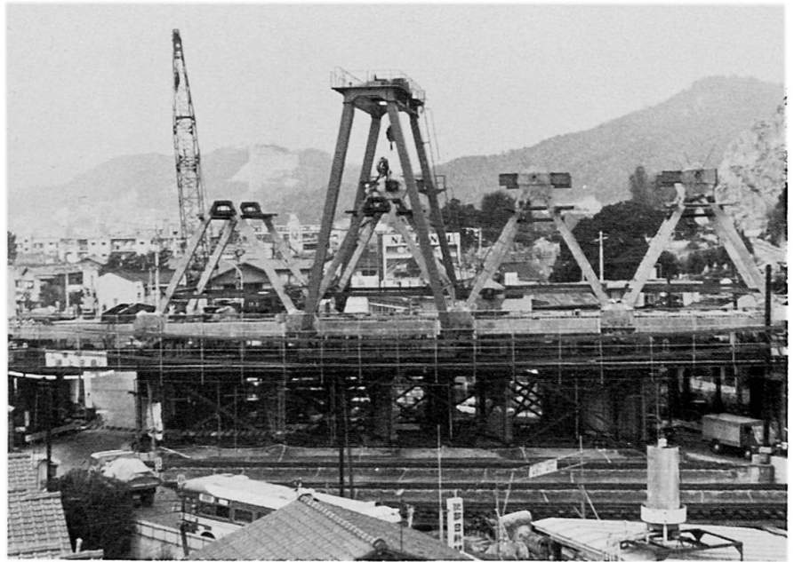
Photo 2. The Iwahana Bridge, erected on the staging
