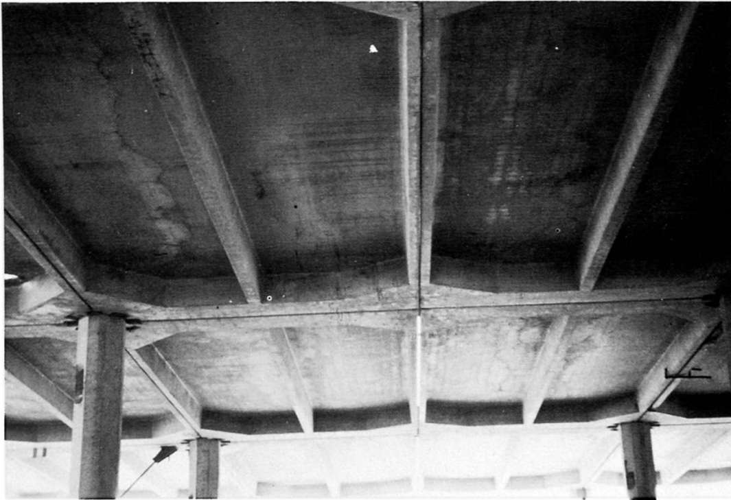
Fig 1: Bottom view of slab elements. At the center of the span, the joint where the elements are coupled is visible.
