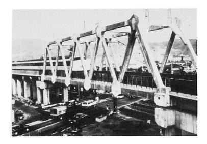
Fig. 1 — Concrete truss bridge of Sanyo super-exress line.
