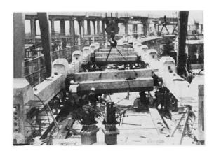
Fig. 2 — Connection of floor beams for truss bridge.
