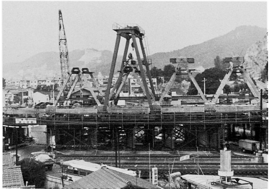
Photo 2. The Iwahana Bridge, erected on the staging
