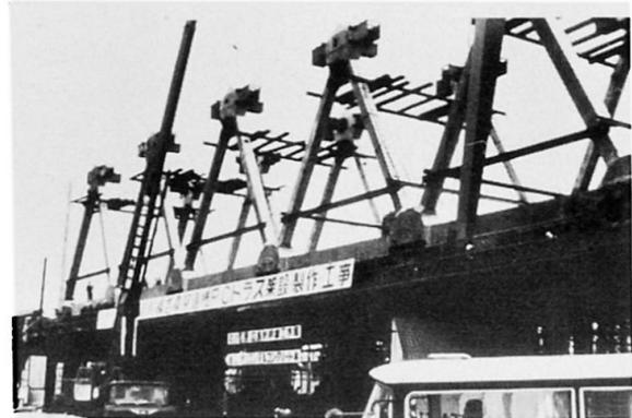
Fig. 3 — Assembly of upper chords for truss bridge.
