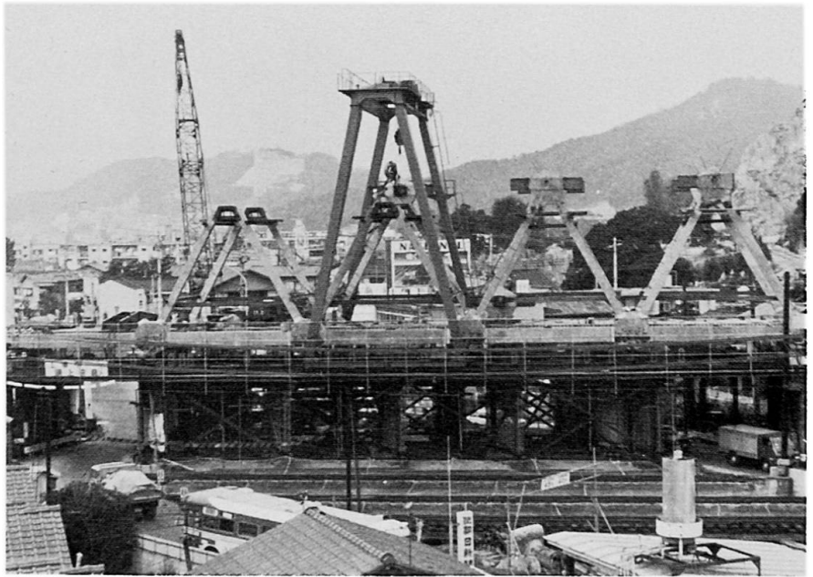
Photo 2. The Iwahana Bridge, erected on the staging
