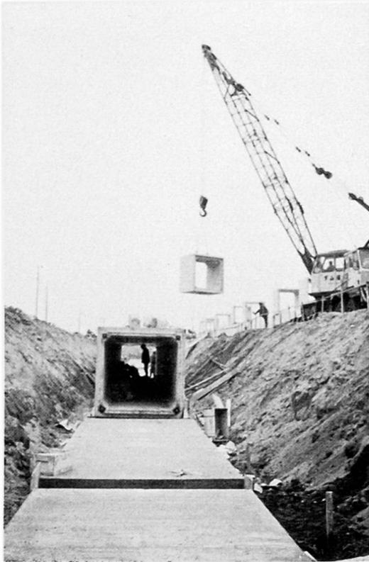
Fig.1 Precast concrete box culvert
