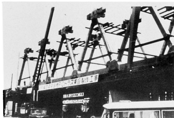
Fig. 3 — Assembly of upper chords for truss bridge.
