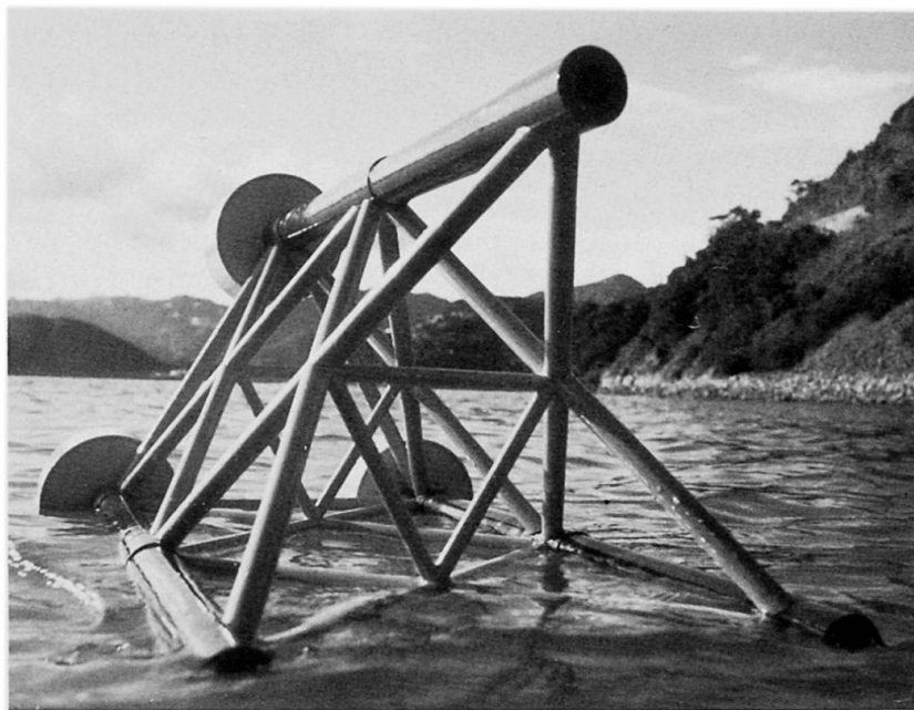
Fig 3. TRICON IS FABRICATED & FLOATED HORIZONTALLY
