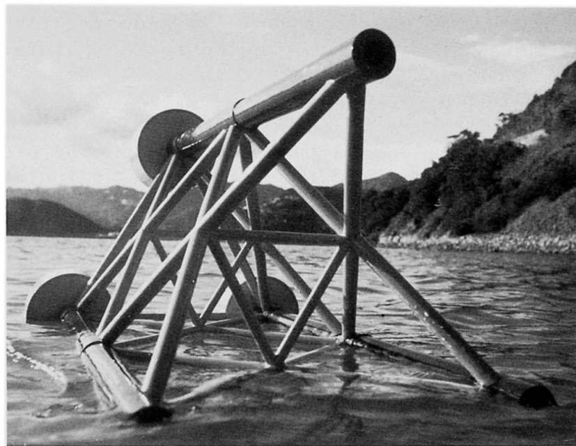
Fig 3. TRICON IS FABRICATED & FLOATED HORIZONTALLY
