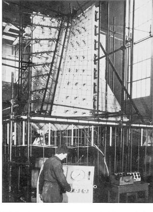
FIG. 6 1:15 scale structural model of the new Cathedral in San Francisco, California, USA, designed by P. L. Nervi. The model is ready for tests to failure.
