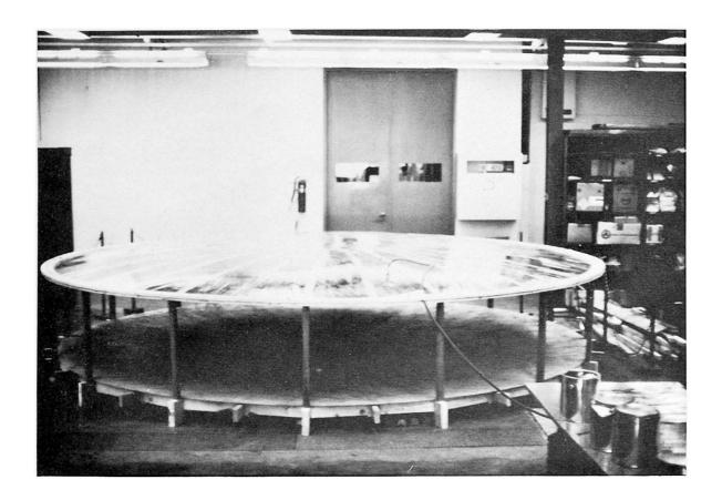
Fig. 4. Model Test of Stainless Steel Balloon Roof. International Nickel Co., New York, N.Y.
