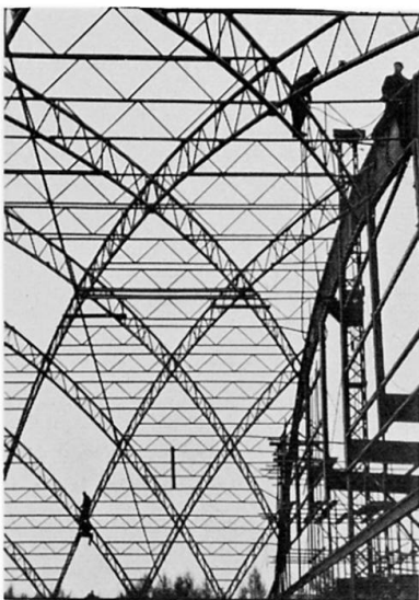
Fig. 9. Erection of a braced barrel vault at Kladno, Czechoslovakia
