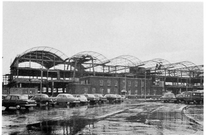
Fig. 8. The external view of seven barrel vaults built for the Port of London Authority
