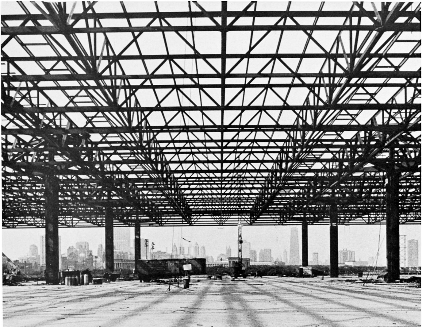
Fig. 1. Two-way latticed grid over the McCormick Plate in Chicago
