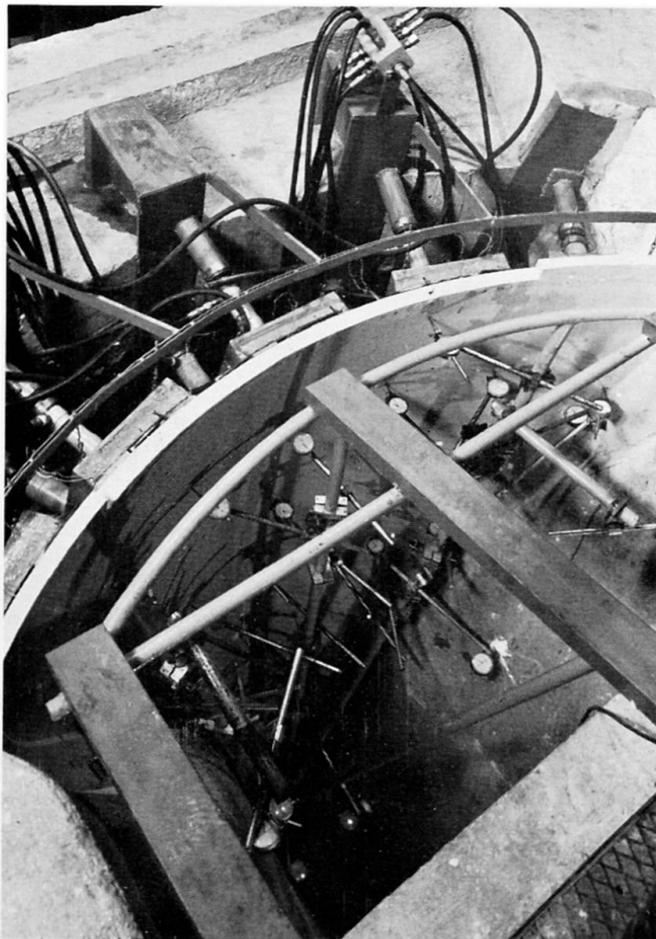
Fig. 14 Vajont Dam. Model under asymmetric load test.
