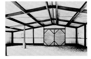
Fig. 9. Roof Truss of Cold-Formed Steel
