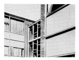
Fig. 7. Exterior Curtain Wall Panel
