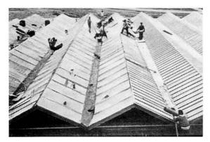
Fig. 21. Hyperbolic Paraboloid Roof Structure
