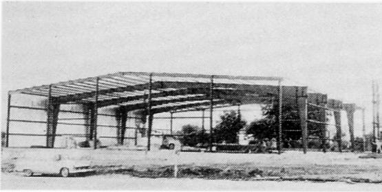
Fig. 11. Standard Building with Cold-Formed Girts, Purlins, Roof and Wall Panels
