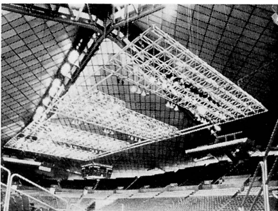
Fig. 17. Space Frame. Lighting Support
