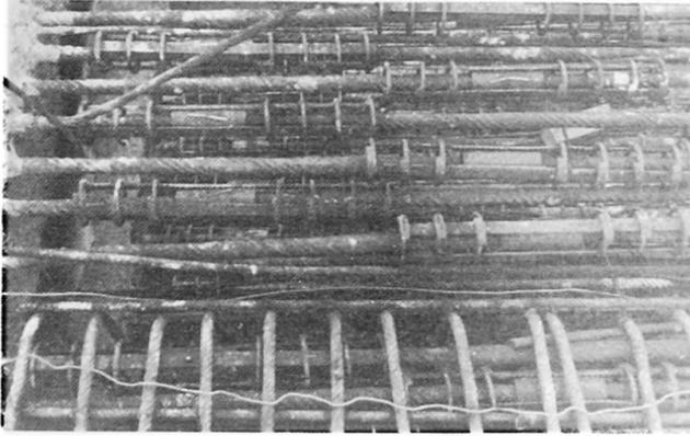
The FY-coupler is a special type of screw-threaded coupler which was developed by the author's team and experimentally tested to secure the transmission of the entire strength of the bar to be joined (12).
