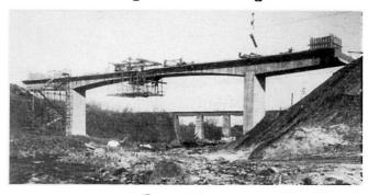
22. The effect of delayed deformation of concrete as well as that of uplifts caused by removal of the counter weights after closing are to be taken into account for the static calculation.
