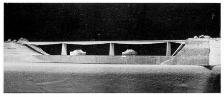
is somewhat larger than 200 m. A bridge built with the new type of structure presented here can lead to a successful bidding when the span of the bridge varies between 150 m and 450m, providing this way a wider field of use for the concrete beam.
