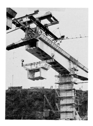
Fig. 10. Single-beam railway bridge at Margecany.
