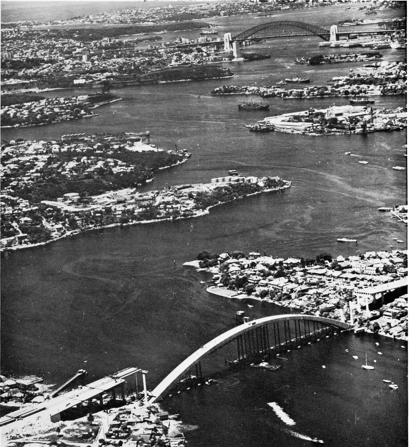
Fig. 8: Sydney Harbour and Distant Pacific – 2 ribs completed
