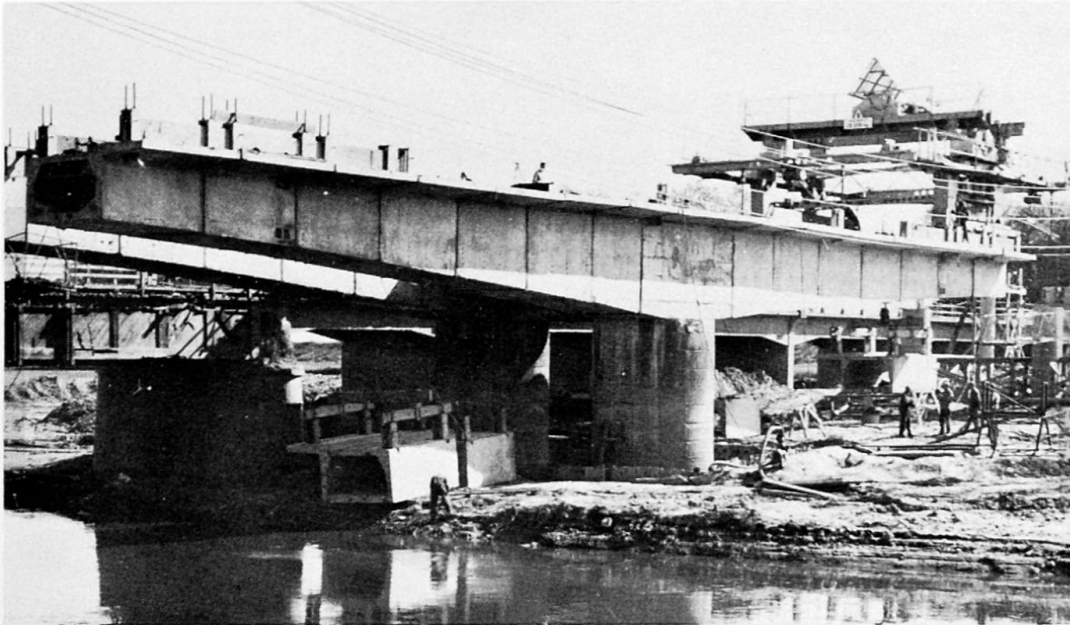
Fig. 7. Half of the Sirník bridge shortly before its completion.
