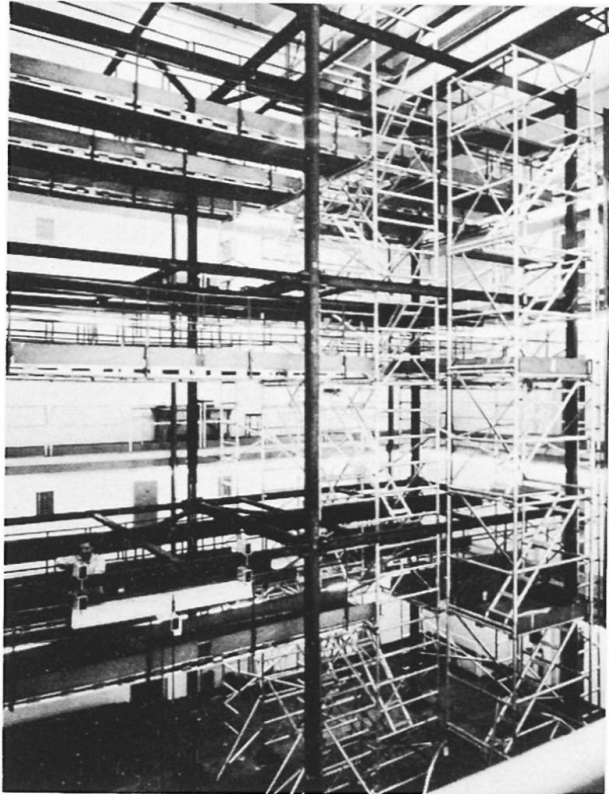
Fig. 4 - Overall View of Test Frame
