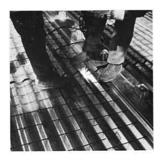
Fig. 8. Category I Form — Closeup showing form being fastened to structural frame.
