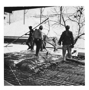
Fig. 10. Category I Form — View showing placement of concrete.
