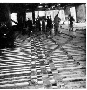
Fig. 12. Category II(b) Form — View showing raceways for wiring with uniformly spaced service fittings.
