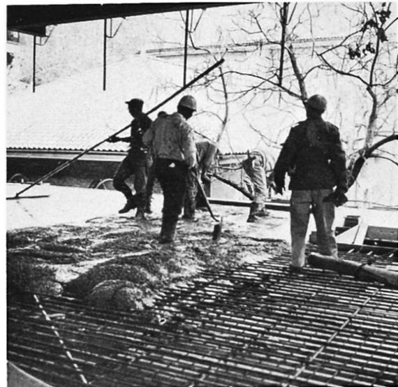
Fig. 10. Category I Form — View showing placement of concrete. (Note negative reinforcing bars.)
