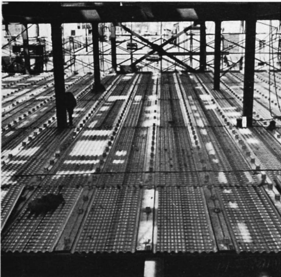
Fig. 9. Category I Form — Overview showing all forms and raceways with service fittings in place.
